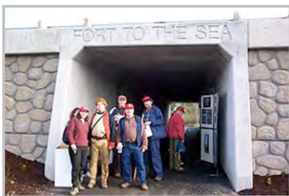
U.S. Highway 101 underpass. The underpass is located two miles from the west end of the trail. (Courtesy the National Park Service)
